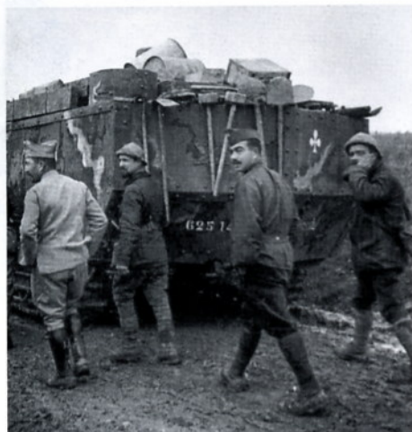
Enlargement from a 45 x 107mm glass view, "Gros Tank Francais." What may look like a garbage truck is actually the rear of a St. Chamond tank in use as a transport vehicle, clearly showing the long overhang.
